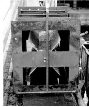
Figure 4. The cathode mounted inside of the box girder.
