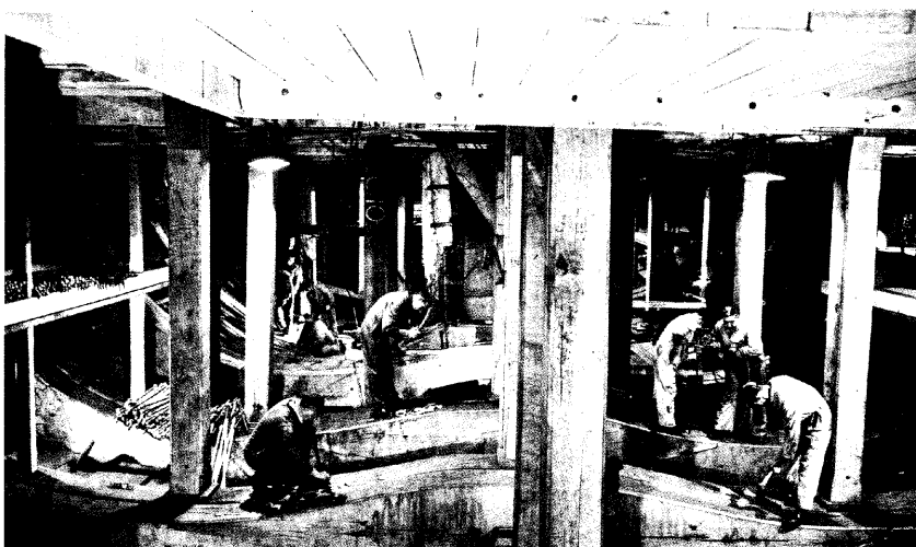
11. Photo of the main hold taken from the forward platform, looking aft. The massive riders are being re-bolted during restoration (taken 25 October 1963). The size of the hold is demonstrated by the men in the photo. The plank structure at the top of the photo is the forward hanging magazine. CPL
