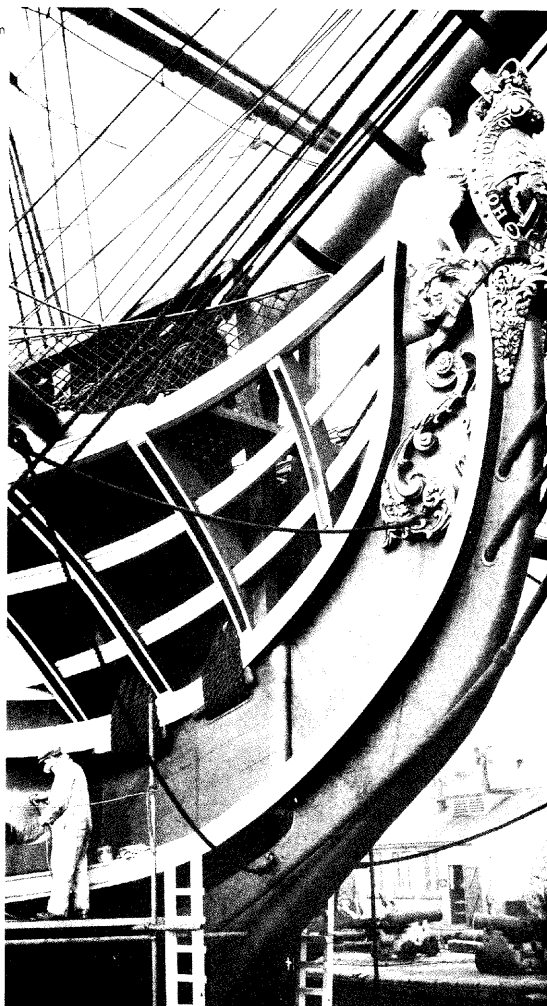
6. Detail of figurehead and head rails. The scale of the ship is demonstrated by the man working on the staging (taken 18 March 1954). CPL
