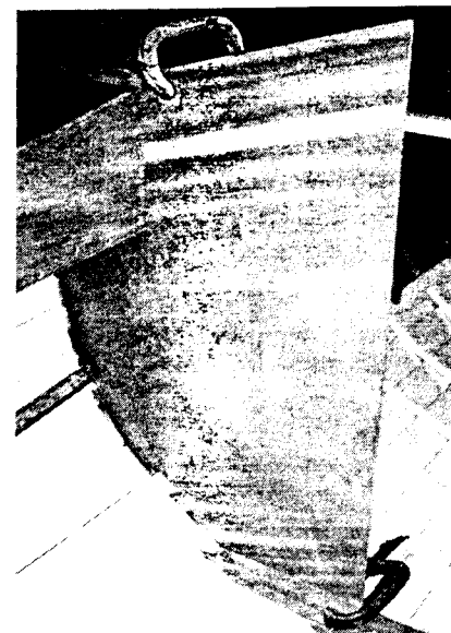
Plate 1.8 The spile board is then removed and the shape transferred to ply.
