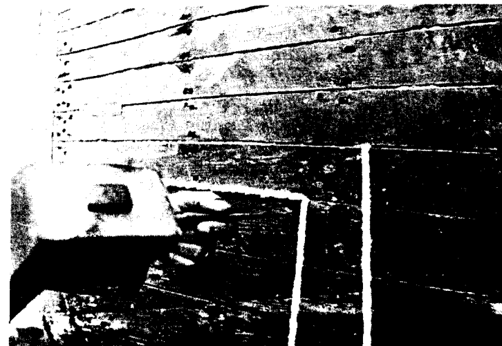
Plate 2.7 Caulking: first a bight of cotton is driven into the seam every 2 in (50 mm).
