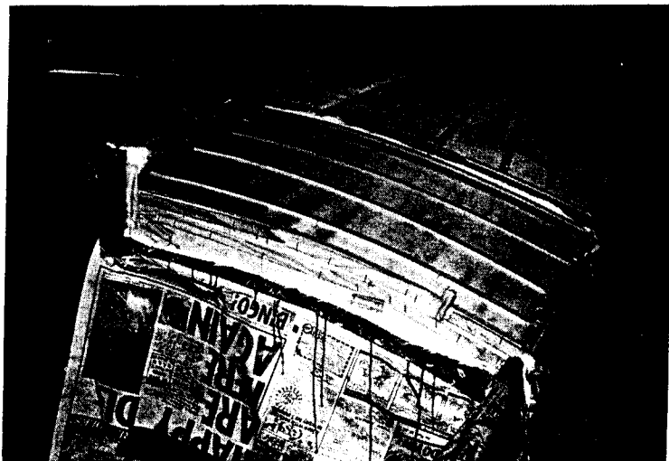
Plate 2.11 Using a Formica 'scraper' over the cloth, the glue beneath it is stretched over as large an area as possible, usually twice that initially painted with glue. Stapled battens then hold the cloth in position until the glue has cured.
