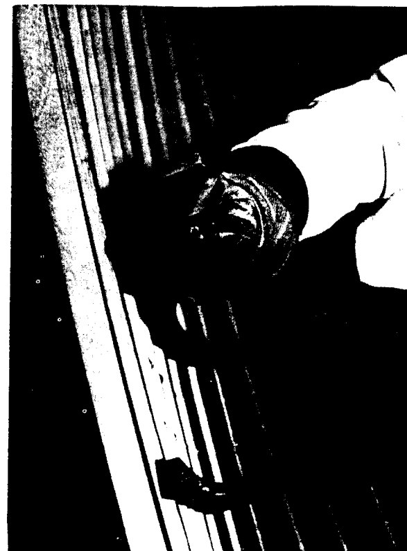
Plate 1.54 Twisting the timber when positioning helps it to accommodate the greater bevels found at the ends of a boat.
