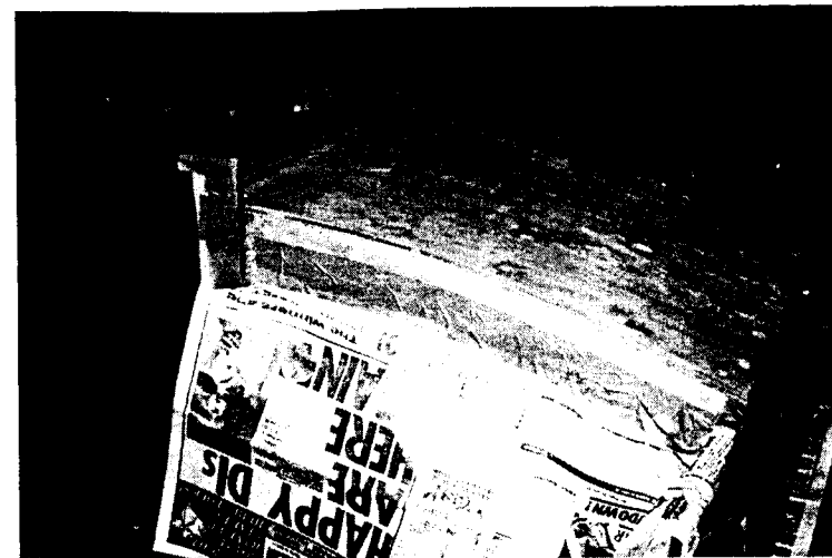
Plate 2.9 'Cascover' sheathing Tirrick's coach roof: the surface is prepared by filling, sanding and wiping clean. Tape is used to mark the limits of the area to be sheathed and newspaper protects other surfaces from dripping glue.
