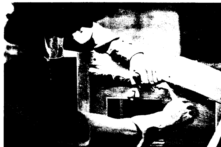
Plate 2.15 Edges are best cut after the timber trim has been fastened in place.
