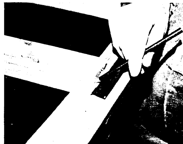
Plate 1.24 Dovetail housing. With the beam slotted into the homelet the dovetail shape is marked.
