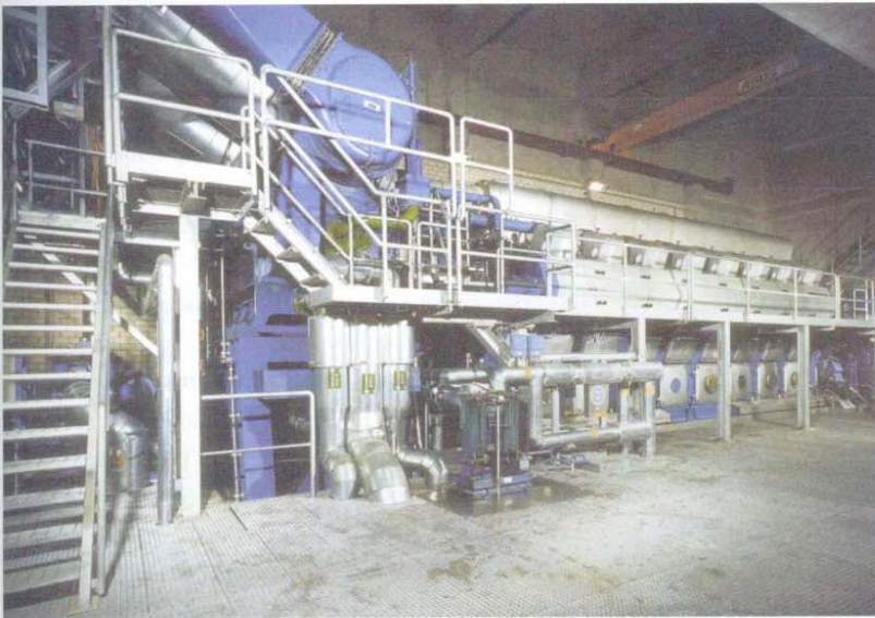
◀ A diesel power plant with a engine running on heavy fuel oil.
