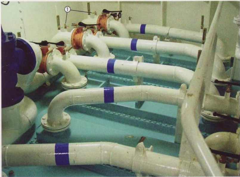
◀ The top view of a box-cooler series. The connections with the various cooling systems are always made on the top side and provided with cut-off valves. Note the vent cocks at the highest point of the piping on the left hand side. 1 vent cocks
