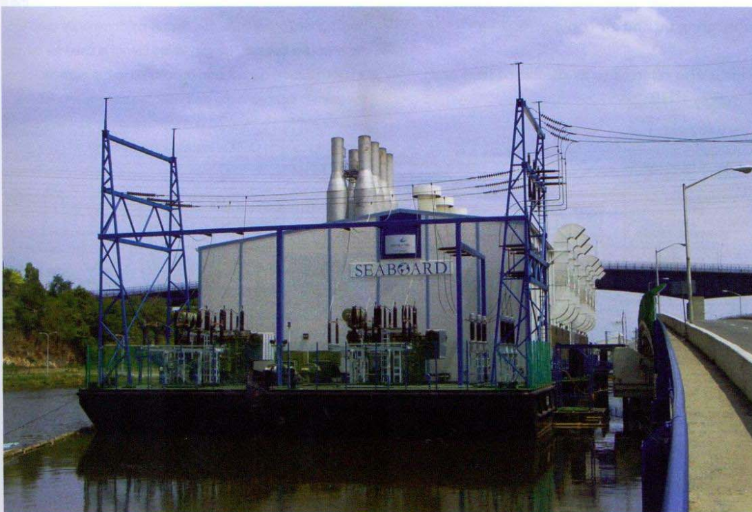
◀ The 'Powerbarge Seaboard' as seen from sea. Eight Wärtsilä-38 engines with eighteen cylinders in V-arrangement generate electricity.
