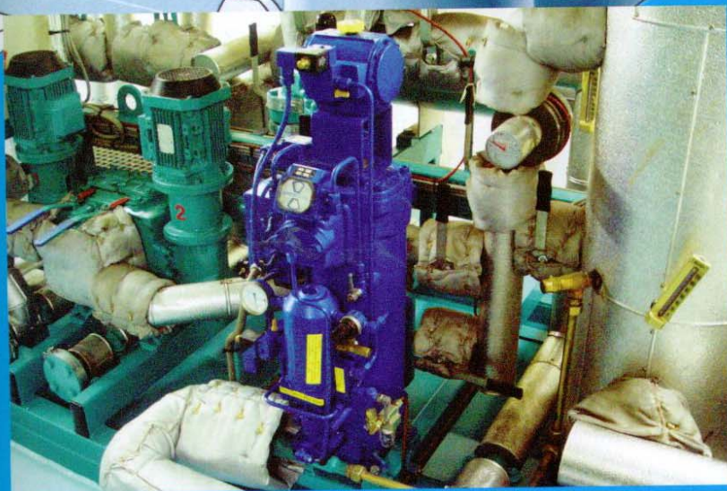
A 'booster unit' with an automatic back-flushing fine-filter.
