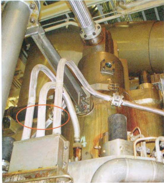
▲ The double-walled high-pressure fuel and lubricating-oil pipe for opening the exhaust valves and the three injectors of a two-stroke crosshead engine.
