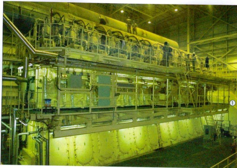
A large two-stroke crosshead engine of MAN-B&W for generating electricity.
