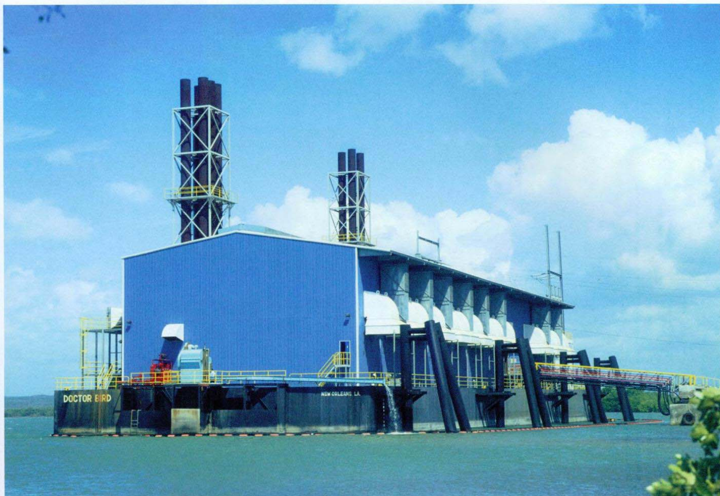
▲ A large floating power plant in the river mouth with Wärtsilä medium-speed diesel engines running on heavy-fuel oil.
