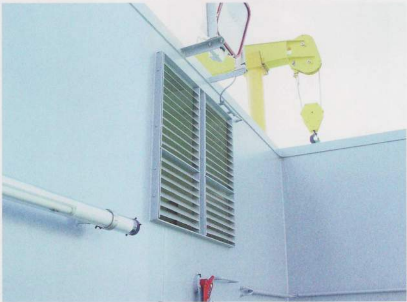
◀ Diesel engines use large amounts of air in the combustion process.
