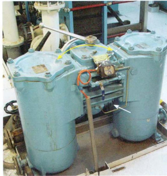
◀ A readily accessible heavy-oil fuel filter. The heavy-oil can be easily led from the one to the other filter element; it is also easy to see when the filter is dirty.
