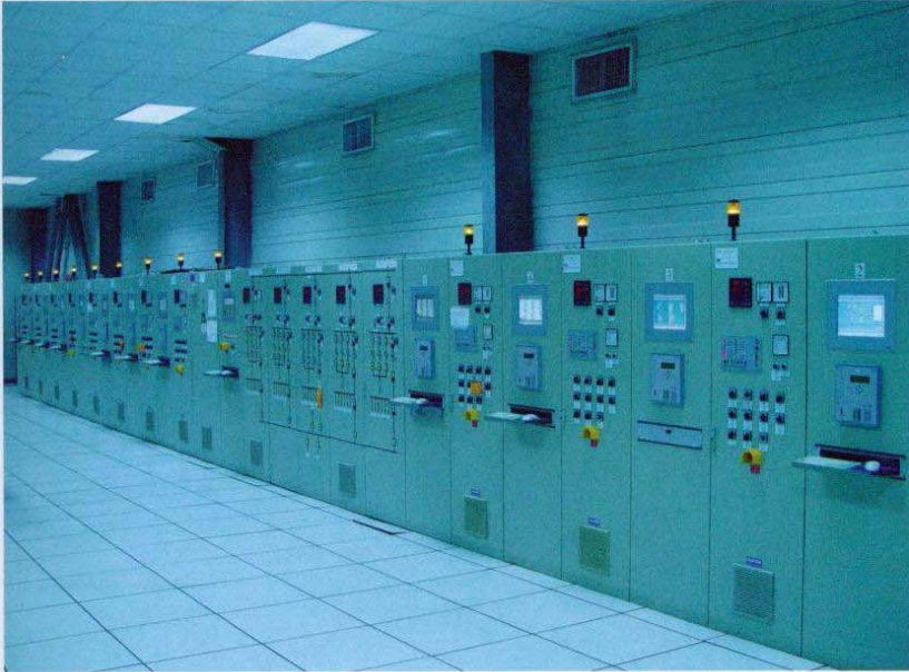
◀ The electric main rail to which all engines are connected.
