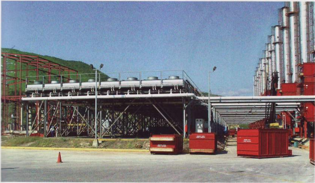
◀ Air coolers in a large diesel-power station in Honduras.
