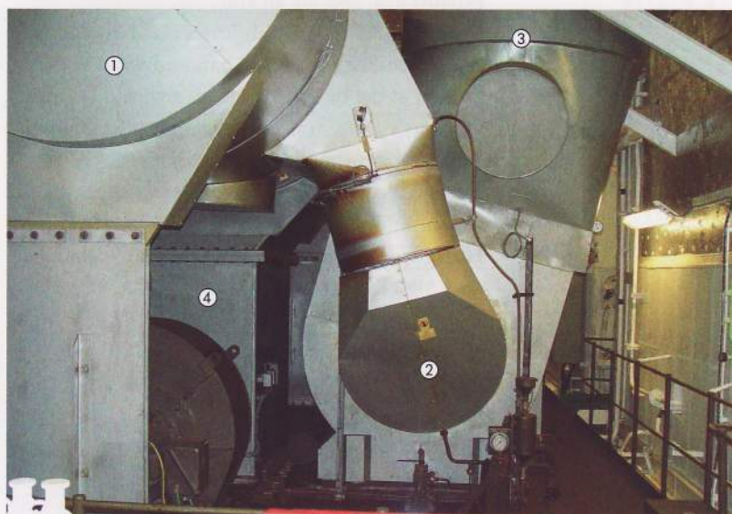
◀ A relatively small diesel genset with turbo-charging.
