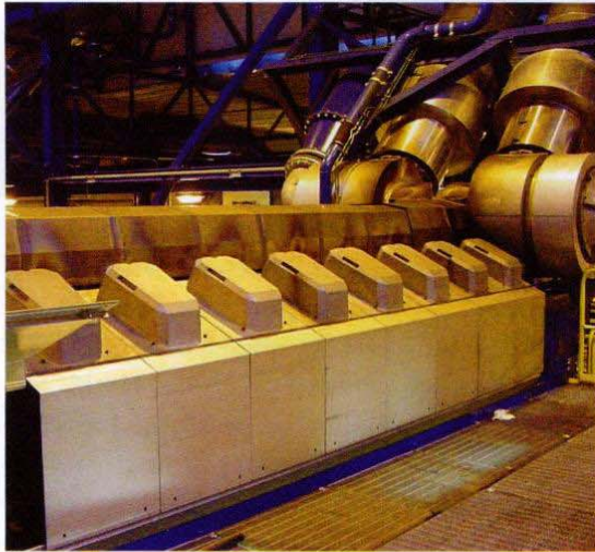
▲ In diesel-power plants, four-stroke medium-speed diesel engines are often used.
