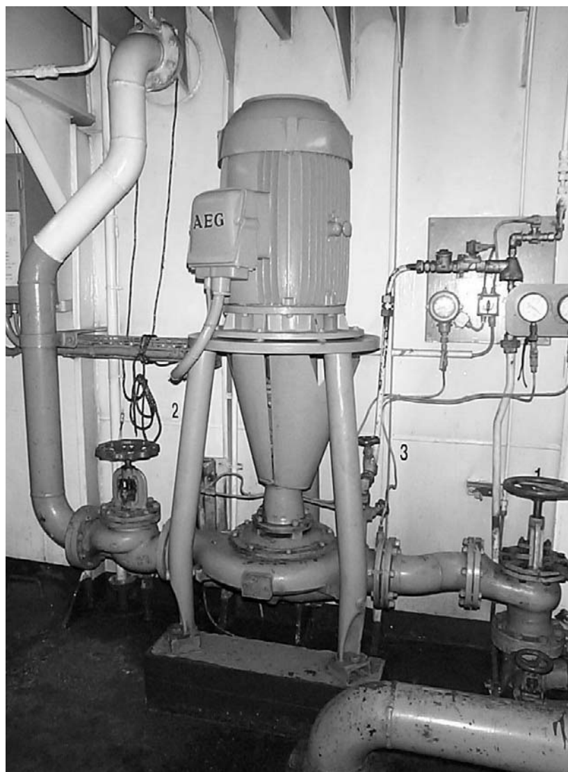
Figure 12 A vertical electric-driven centrifugal water pump
