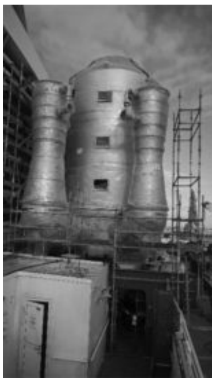
Figure 43. Installation of the exhaust gas scrubber on Allure of the Seas.
