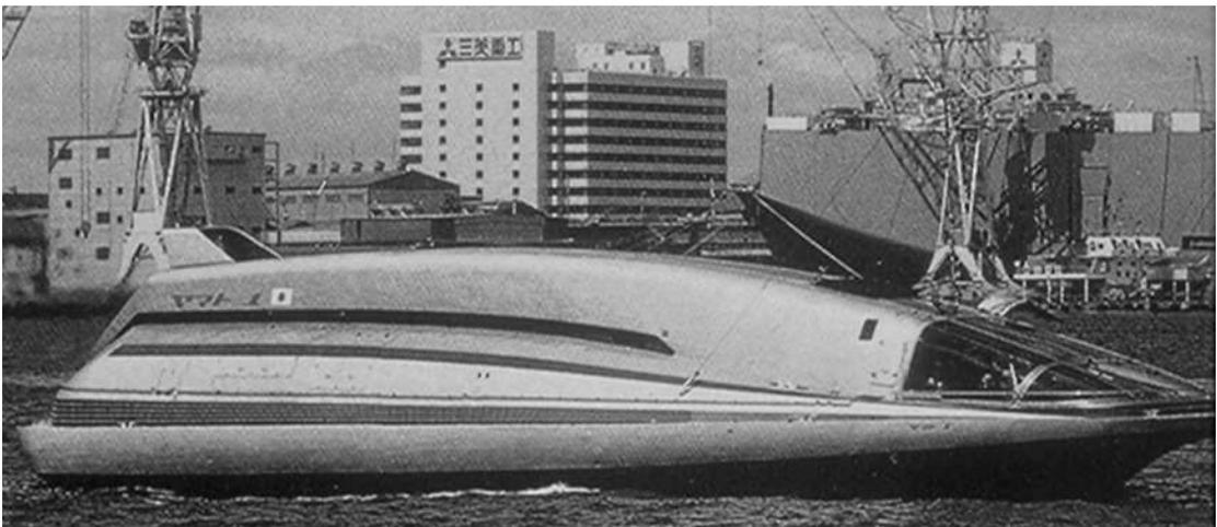
**Figure 2.19** *Yamato 1*: Experimental magnetohydrodynamic propulsion craft
