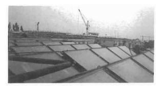
Figure 12.6 Flat-plate collectors on the roofs of blocks of flats in Bucharest
