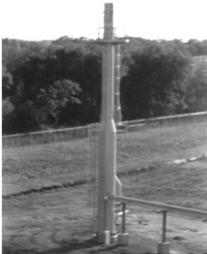
Figure 12-1. Flare stack. Courtesy Nisseki Chemical Texas, Inc., Bayport, Texas.
