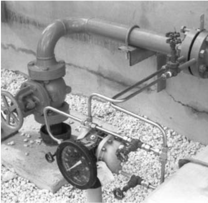
Figure 12-7. Orifice flanges with valve taps. Courtesy Nisseki Chemical Texas, Inc., Bayport, Texas.
