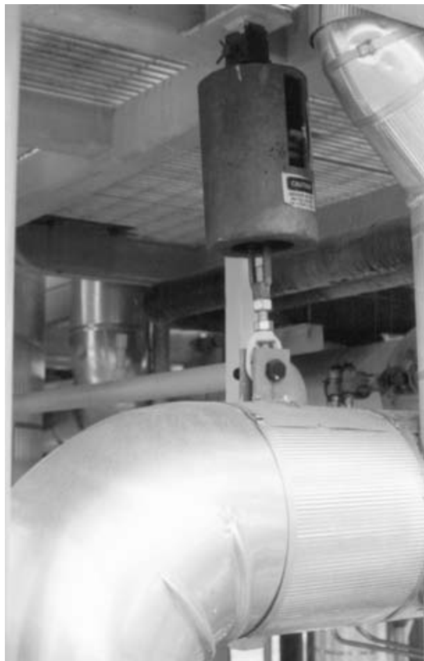
Figure 11-18. Spring hanger. Courtesy Nisseki Chemical Texas, Inc., Bayport, Texas.
