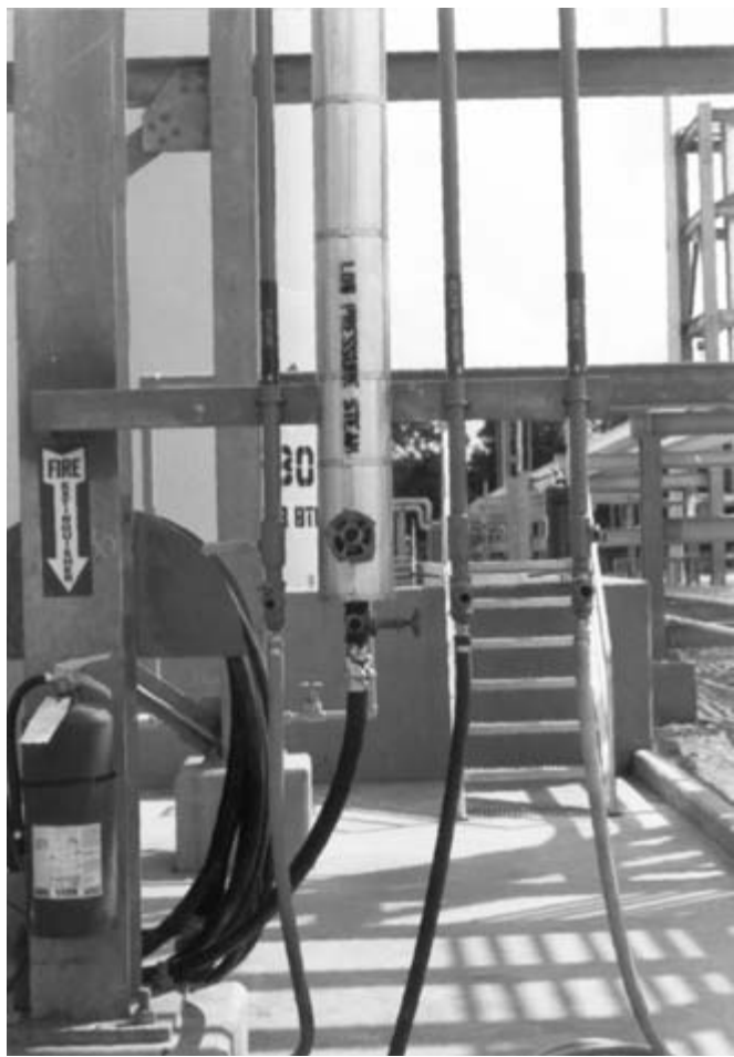
Figure 12-5. Utility station. Courtesy Nisseki Chemical Texas, Inc., Bayport, Texas.
