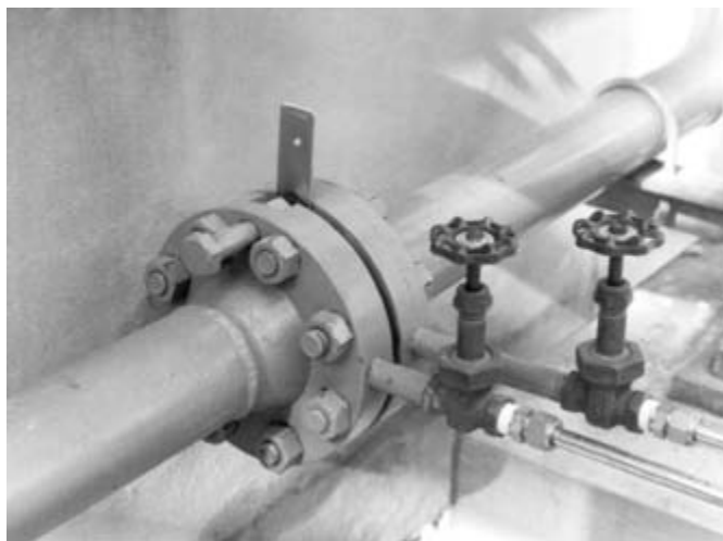
Figure 4-26. Orifice flange union assembly. Courtesy of Nisseki Chemical Texas Inc., Bayport, Texas.
