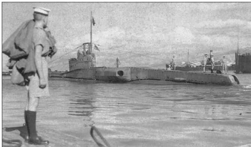
Traveller returning to Beirut on 1 October 1942. This photograph shows the other major modification to the Group 2 'T' class boats which was to reverse the midships external tubes so that they faced aft. With the addition of a single stern tube under casing, this gave a stern salvo of three torpedoes. Traveller was lost, presumed mined, in the Gulf of Taranto on or around 4 December 1942. The seven Group 2 'T' class boats all served in the Mediterranean where five of them were sunk.
