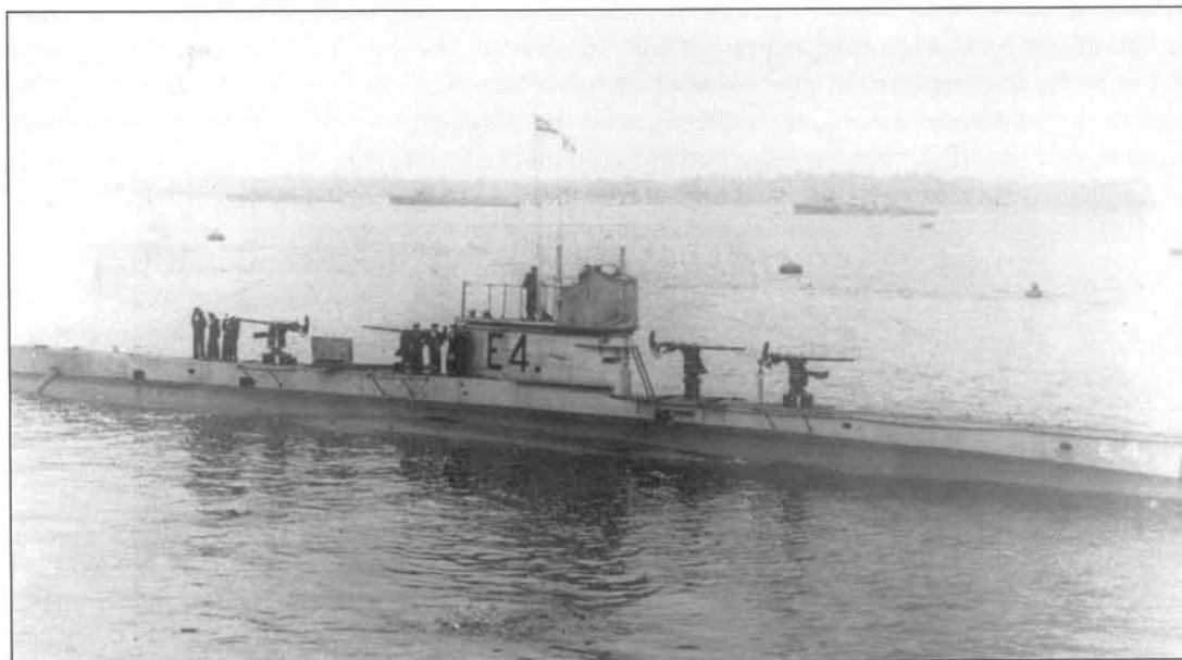
E.4 at Harwich in the early days of the war with an unusual armament of four 6 pounders on high angle mountings, a sure sign that German Zeppelins were making their presence felt. The gun was to play an important role in submarine operations, both as a means of self-defence and as a weapon used to sink small targets not worth a torpedo. E.4 was commanded by one of the great characters of the early Submarine Service, Lieutenant E.W. Leir, known as the 'Arch Thief' who plundered His Majesty's Navy of anything portable and of whom it was said that only his DSC was earned honestly! E.4 was subsequently lost with all hands in a collision with E.41 on 15 August 1916.
