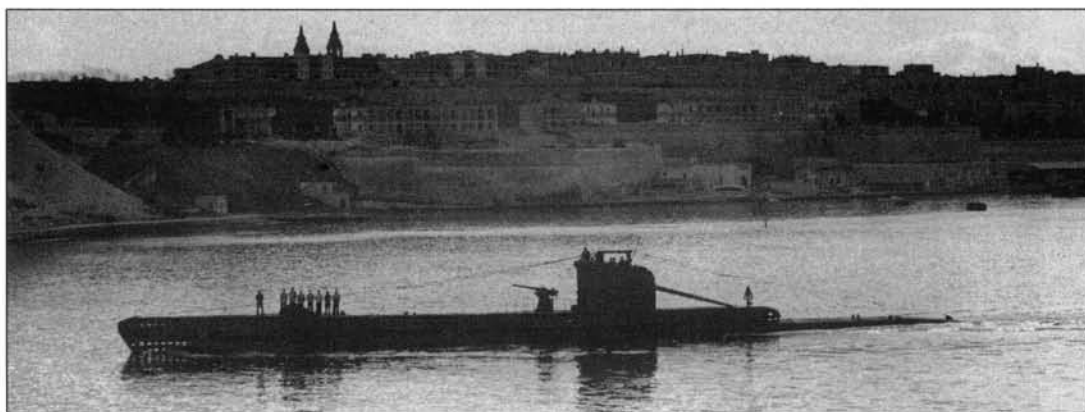
HMS Una at Malta on 13 February 1943. Una and Umpire were built by the Royal Dockyard at Chatham whereas all the remaining forty boats were built at Barrow by Vickers. Note the shape of the bow compared to Ursula . The large lump on the bow made by the two external torpedo tubes provoked a number of complaints, namely that it reduced speed and caused a noticeable wave on the surface when the boat was running at periscope depth. As a result the two external tubes were removed and the bow lengthened and flattened. However, Upholder , Unique , Upright , Usk , Utmost and Unbeaten were too far advanced in their construction to be thus modified. As a result they retained the raised bow but were not fitted with external torpedo tubes. Una enjoyed a varied career in the Mediterranean (see Eric Newby's Love and War in the Appenines for a description of one operation in which she was involved) and then returned to the UK where she was employed in a training role.
