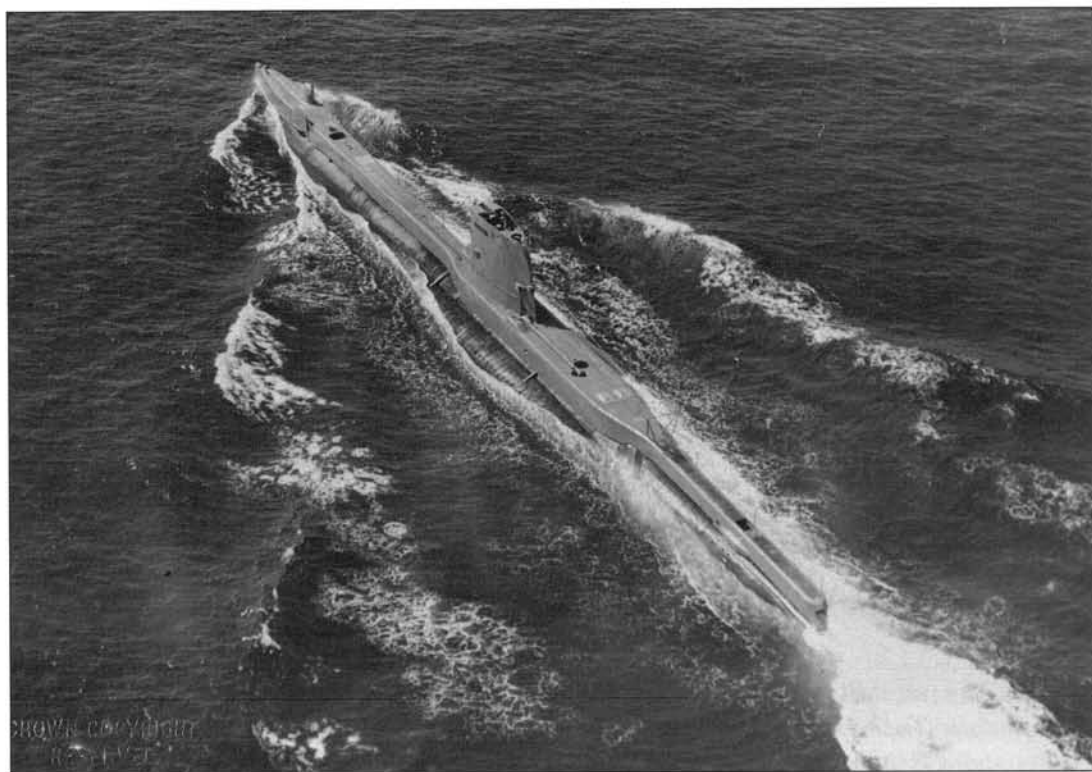
HMS Tireless was one of five T-boats selected for 'streamlining', an economy conversion programme in which the hull and casing were streamlined and a new fin was fitted; no other structural modifications were carried out.
