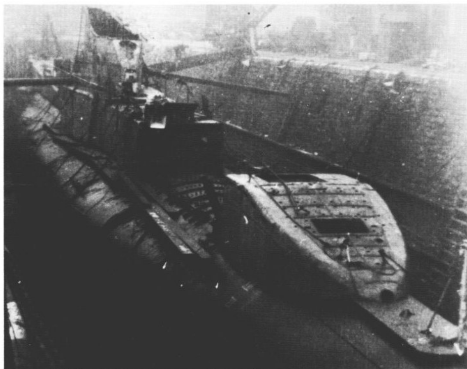
► Job No. 1027, ex-HMS Thetis , in Cammell Laird's dry dock after being raised following her loss during her first dive on 1 June 1939. She was extensively refitted by Cammell Laird before recommissioning as Thunderbolt .
