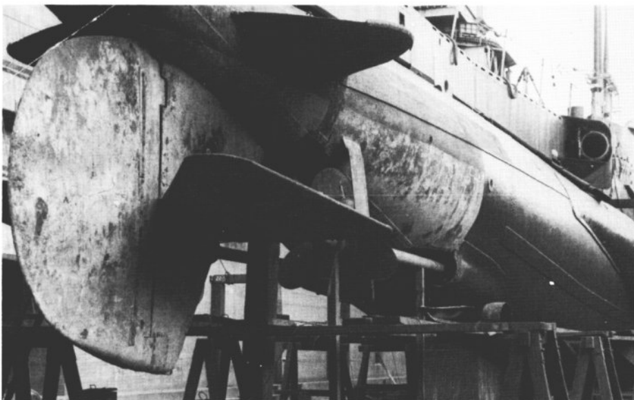
◀ HMS Telemachus in dry dock at Sydney, Australia in 1951, showing the rudder, starboard propeller and after hydroplane. At the top right is an open aperture for No. 9 torpedo tube. (Gus Britton)
