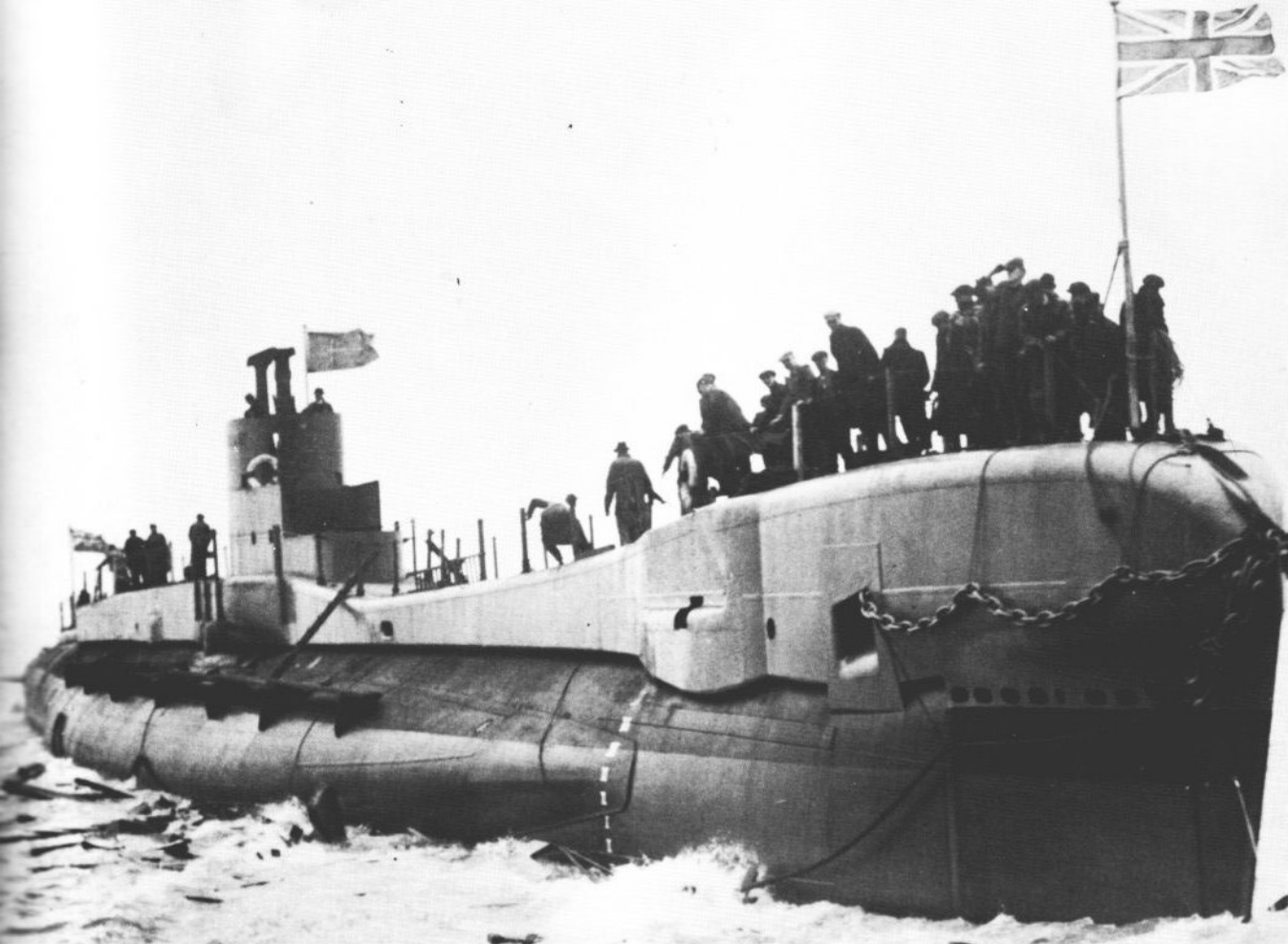
▲ HMS Truant , launched at Vickers' Barrow yard on 5 May 1939. In contrast to Thetis , her periscope standards are erected, but she has not yet been fitted with her 4-inch gun.
