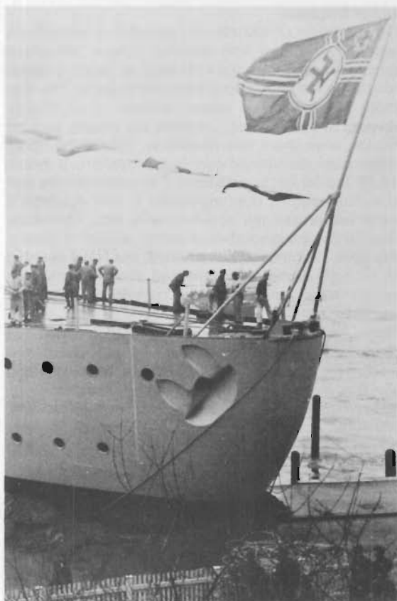
After launching the hull of Gneisenau went out of control and the stern collided with the quayside. Workmen are seen here inspecting the damage to the stern, but damage to the quay is more evident! (Author's Collection)
