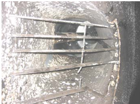
Figure 3 One broken grid
