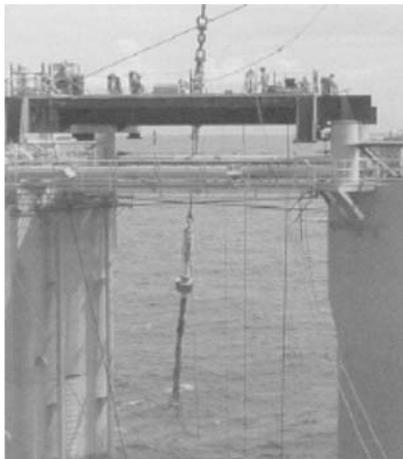
Figure 9.64 The Prince SCR during hang-off installation showing the pre-installed VIV strakes [Gore and Mekha, 2002]
