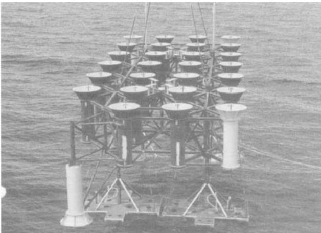
Figure 14.20 Subsea template lifting
