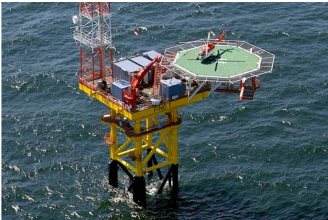
Fig. 4. Platform deck with helicopter pad and containers (Photo: Hero Lang)
