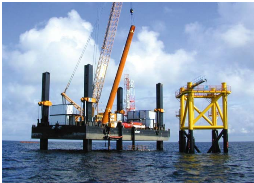
Fig. 2. Offshore working platform with crane and pile. On the right side: FINO 1 platform under construction
