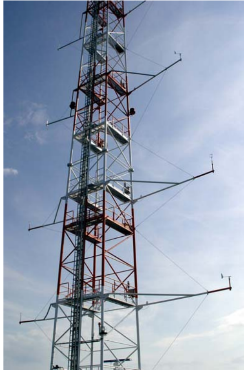
Fig. 5. Wind measurement mast with meteorological sensors (Photo: Deutsches Windenergie Institut, Wilhelmshaven, DEWI)
