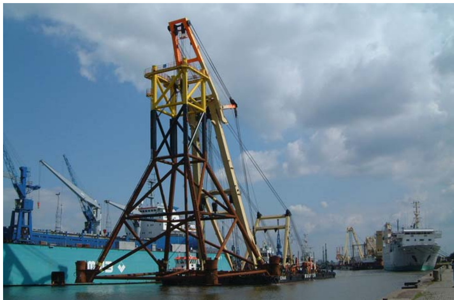
Fig. 6. Transport of the jacket by floating crane (Photo: GL Wind)
