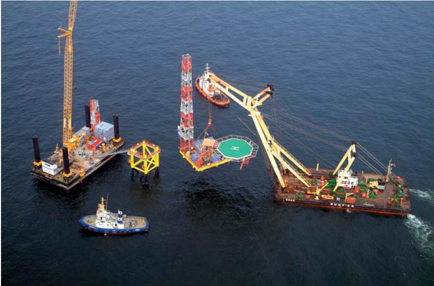
Fig. 7. Lifting operation of the platform deck (Photo: Hero Lang)
