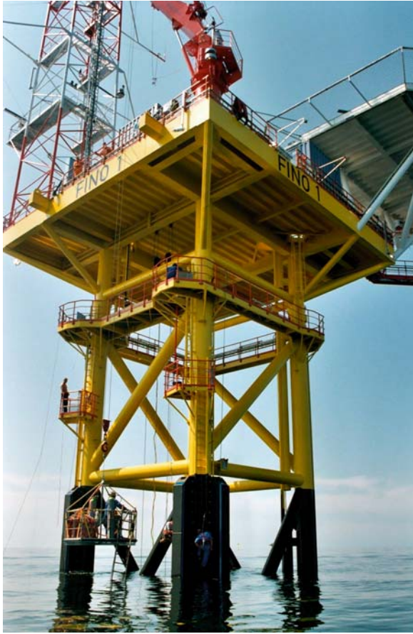
Fig. 8. Maintenance work at FINO 1 (Photo: GL Wind)
