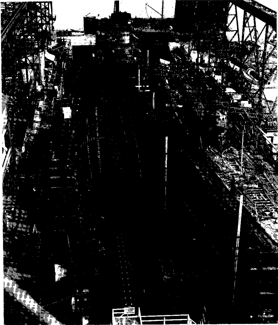
Under construction at Mare Island on 2 January 1941, the submarine Silversides illustrates double-hull construction. The inner circular section is the pressure hull; the framing, which surrounds it, supports a thin streamlined outer hull. Such a configuration leaves the interior of the pressure hull unencumbered by framing and allows for a streamlined outer hull whose shape is not determined by the need to resist water pressure.
