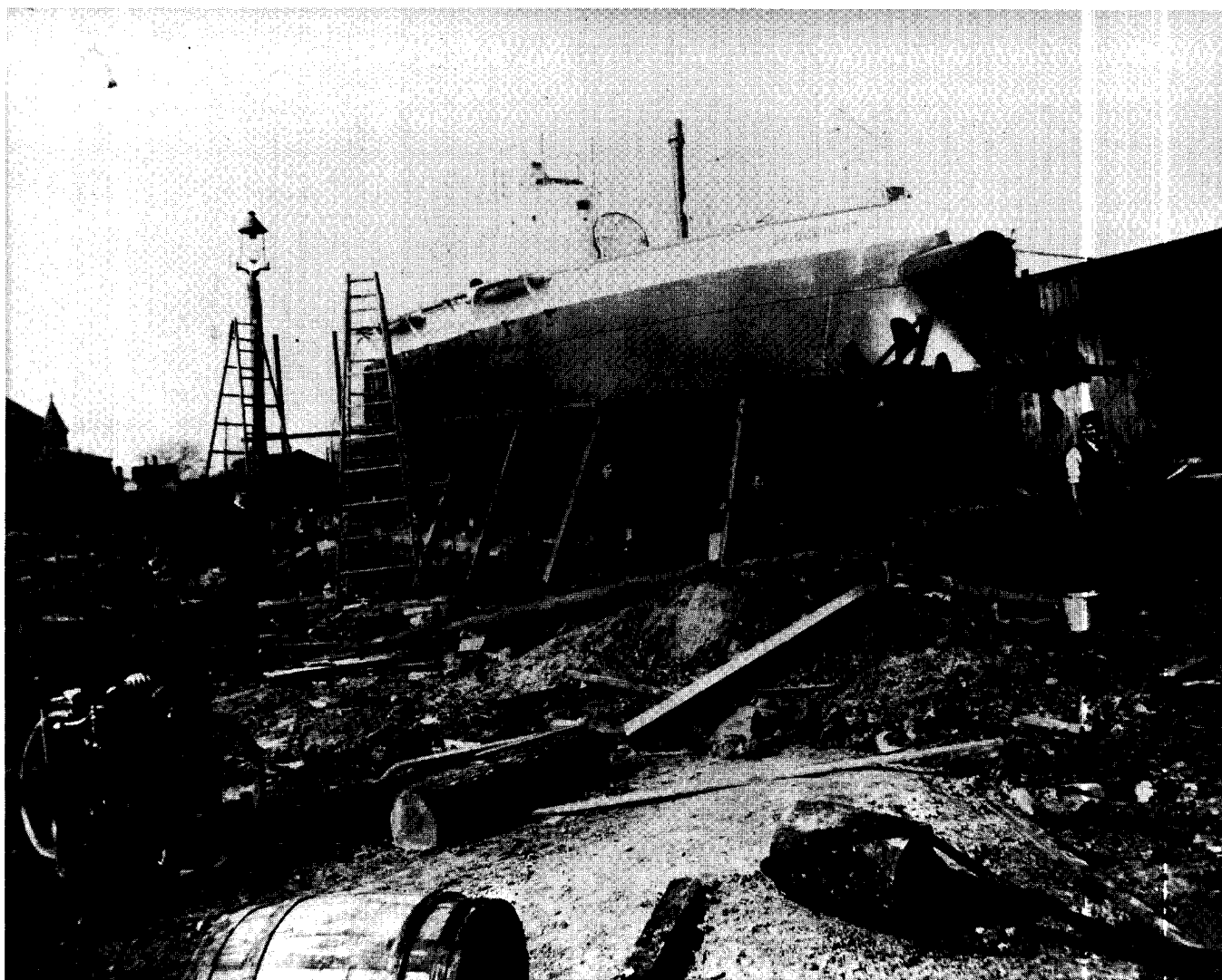
Ready for launch at Bridgeport, Lake's Protector shows his characteristic twin-screw stern and a single after torpedo tube. The two port-side hydroplanes are visible at the deck edge near the conning tower; the pipe farther aft is the engine exhaust. This photograph was taken no more than a month before the submarine was launched on 1 November 1902. (Submarine Force Museum and Library)
