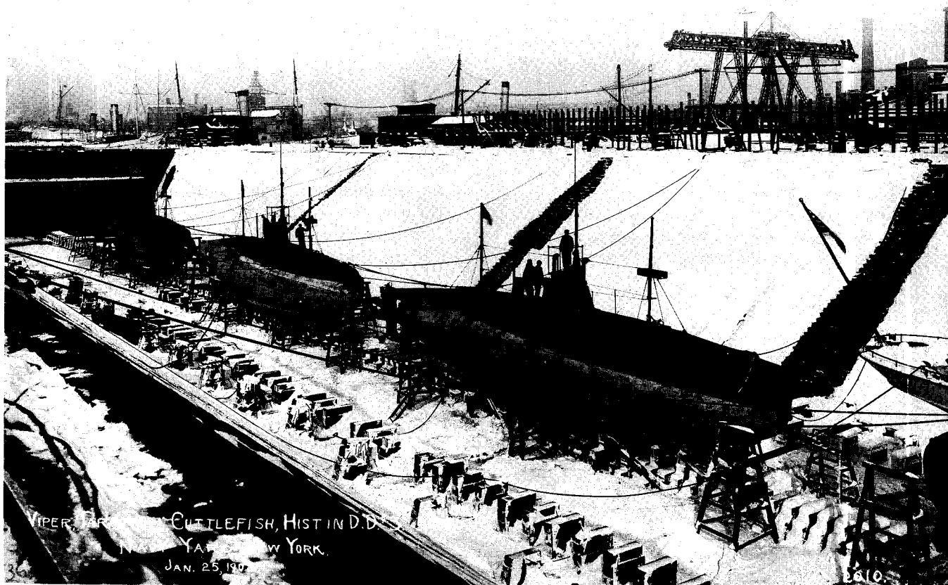
The three B-boats ( Cuttlefish , Tarantula , Viper ) share a snowy dry dock at the New York Navy Yard, probably in 1907. Note that each one still has a single tall fixed periscope, with a flagstaff above it. Boats running submerged flew flags on these staffs to warn surface ships against running them down. Note, too, the running lights affixed to boards on the foremasts. (Collection of Rear Adm. Henry Williams)
