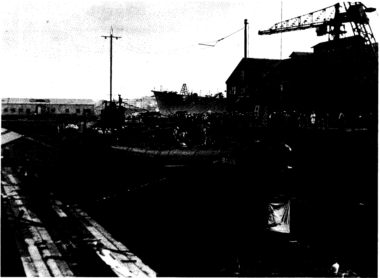
In dry dock in the 1930s, Bass shows her bulbous forefoot (carrying her bow torpedo tubes) and her clipper stem and flared deck. As in many surface ships, the bulbous bow was intended to reduce wavemaking resistance and thus to improve the submarine's surface speed; the unusual bow was expected to make the deck drier.
